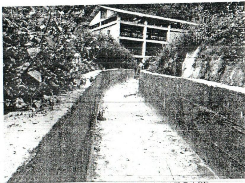
POWER HOUSE BUILDING & TAILRACE
