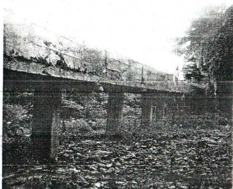
C/O AQUADUCT AT POWER CHANNEL
